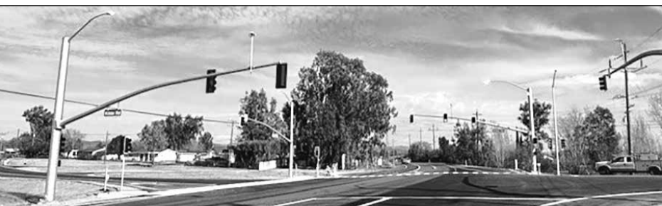
A newly activated traffic signal controls traffic at the intersection of State Route 20 and Kibbe Road in Yuba County. The signal provides direct access to the Hallwood Aggregate Plant and is intended to improve traffic flow and safety while reducing truck traffic on nearby Walnut Avenue. Photo courtesy of Caltrans
