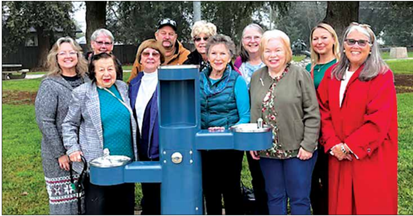
On Jan. 21, a jubilant group of Dixon women joined officials from Dixon Public Works to celebrate the installation of a new water fountain in the Dixon Women's Improvement Club Park, located at the corner of C and First Streets. Photo courtesy of Dixon Women's Improvement Club
