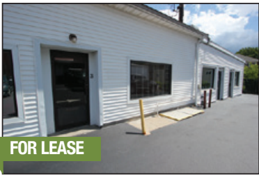
16-3 Cottage St., Franklin 850SF, $1500/mo, Office
