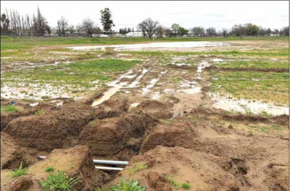
The Feb. 17 findings follow Harden's October report, when a 16-foot test hole sank 11 inches within an hour and deeper drilling revealed more than 20 feet of clean sand. Photo by Seti Long
