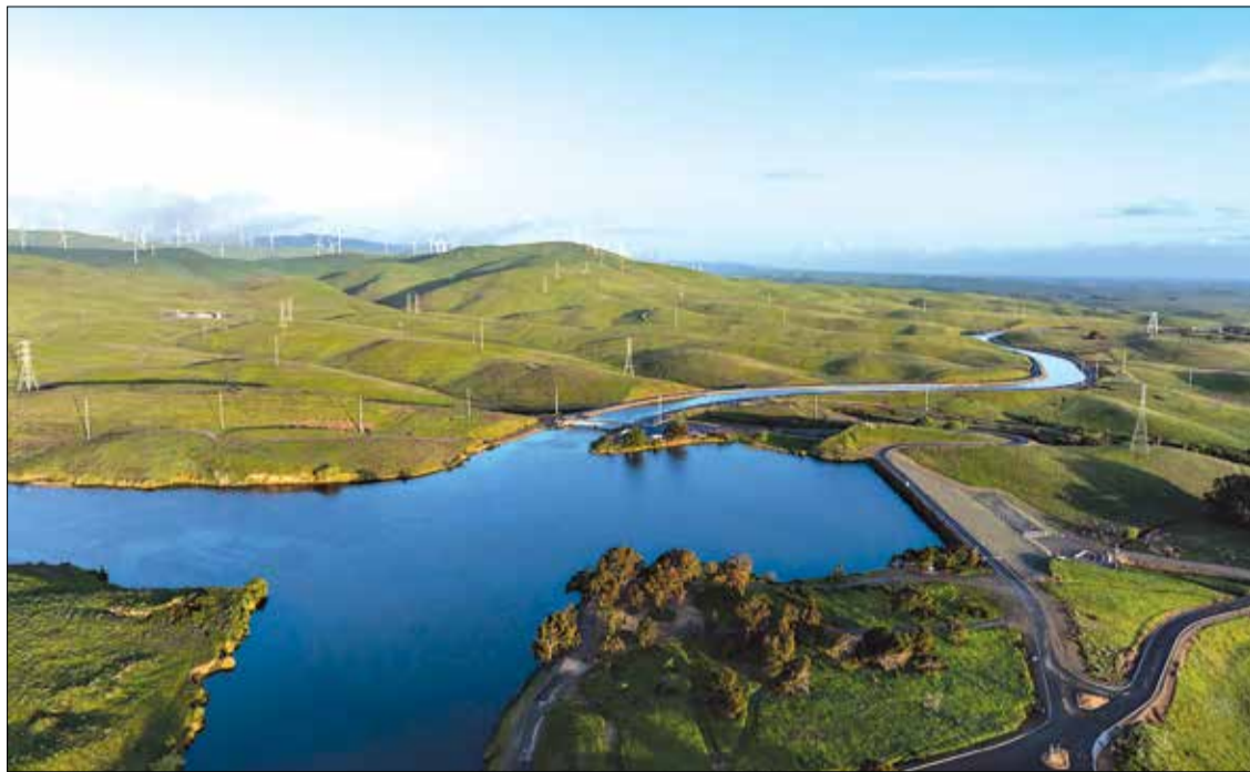
A drone view of the Bethany Reservoir, impounded by five dams in Alameda County, serves as a forebay for the South Bay Pumping Plant and afterbay for Banks Pumping Plant. Photo taken March 28, 2024. Photo courtesy of California Department of Water Resources
