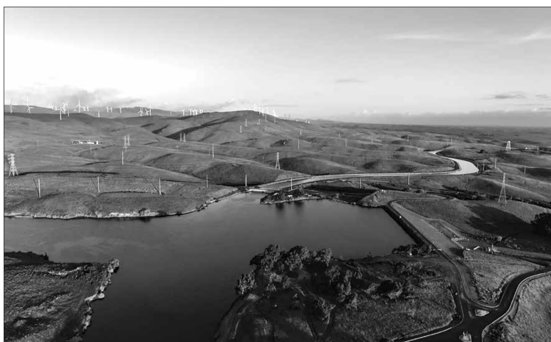
A drone view of the Bethany Reservoir, impounded by five dams in Alameda County, serves as a forebay for the South Bay Pumping Plant and afterbay for Banks Pumping Plant. Photo taken March 28, 2024. Photo courtesy of California Department of Water Resources
