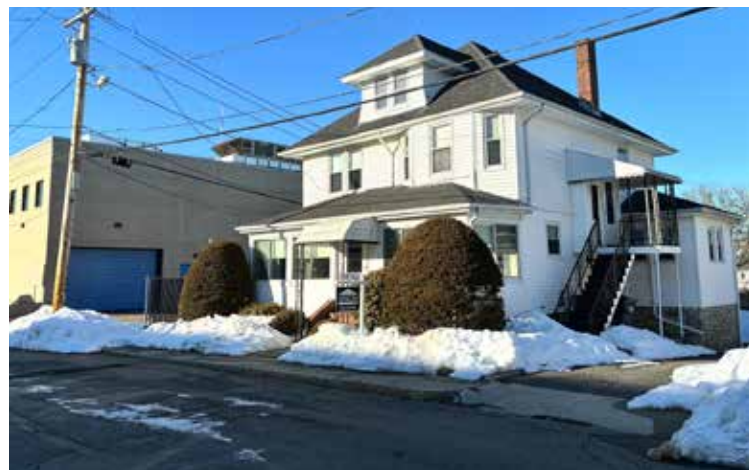
At a Feb. 9 Special Town Meeting, residents voted to take the house at 6 Park Terrace by eminent domain for fair market value ($520,000). The property is sandwiched between two town-owned properties and will be utilized by the police department. Photo credit Theresa Knapp
