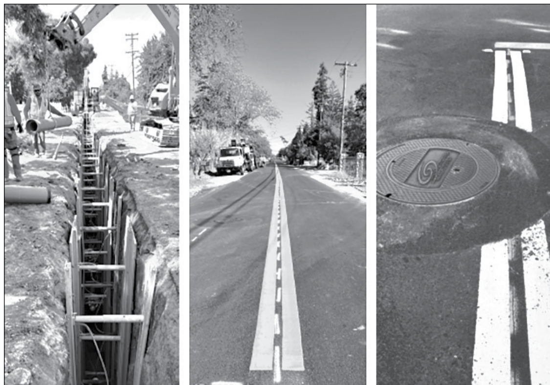
SacSewer connected homes to the public sewer system with newly constructed sewer pipes and manholes, and private septic tanks were safely decommissioned. Photo courtesy of Sacramento Area Sewer District
