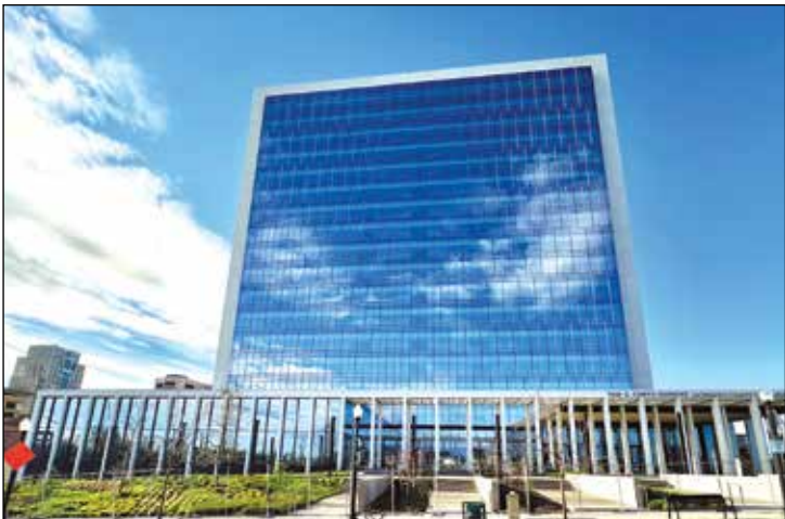
The new Tani G. Cantil-Sakauye Sacramento Superior Courthouse located in the Sacramento Railyards is set to open next month. Photo courtesy of Sacramento County Superior Court
