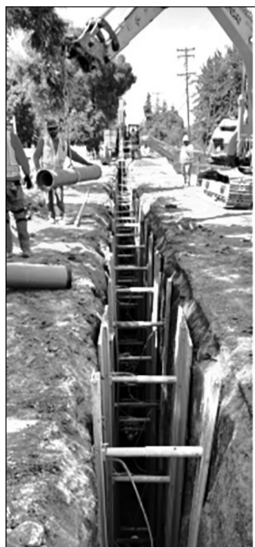
SacSewer connected homes to the public sewer system with newly constructed sewer pipes and manholes, and private septic tanks were safely decommissioned. Photo courtesy of Sacramento Area Sewer District
