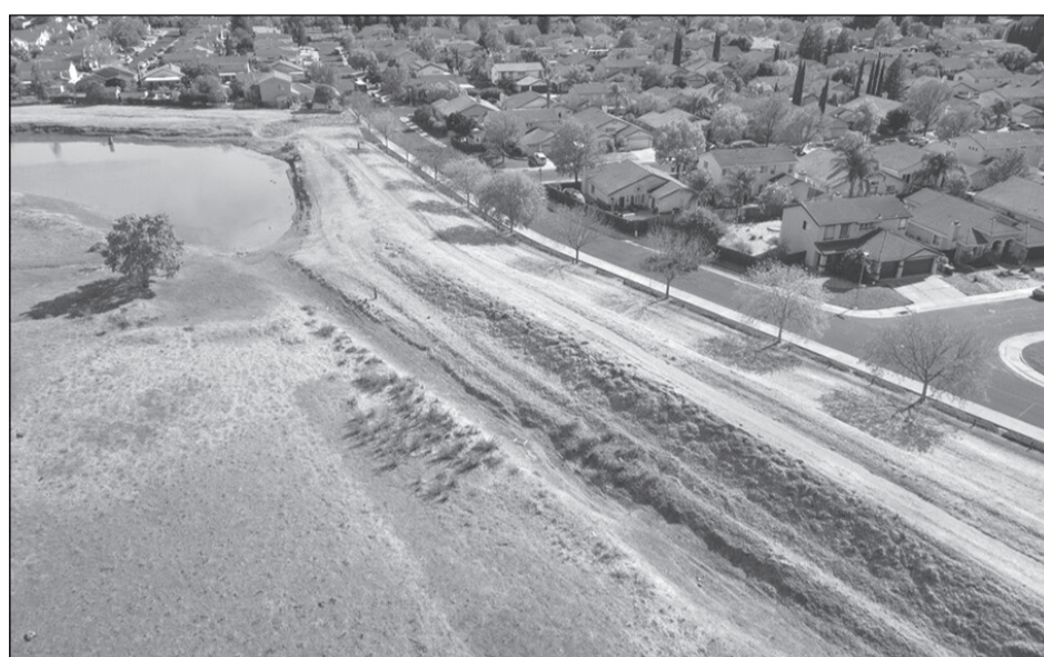
The city announced in its latest newsletter that construction on a multi-use trail segment along Laguna Creek Trail and Bruceville Road will begin this summer, along with a new right-turn lane at the intersection to help reduce traffic. Photo courtesy of City of Elk Grove
