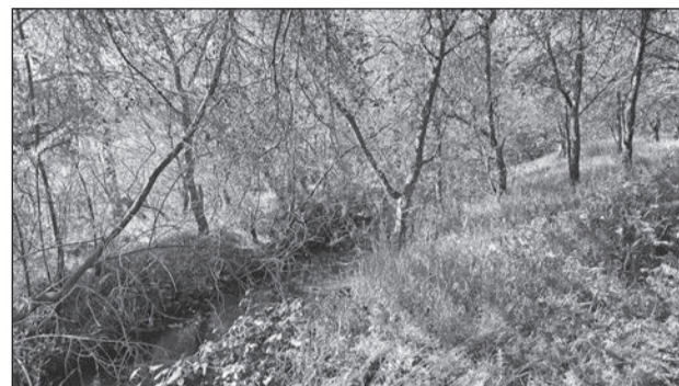
This image shows a section of the CIA Ditch before clearance work began. Photo courtesy of Rancho Murieta Properties
