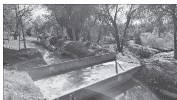
The image shows a section of the CIA Ditch after clearance work was completed. Photo courtesy of Rancho Murieta Properties
