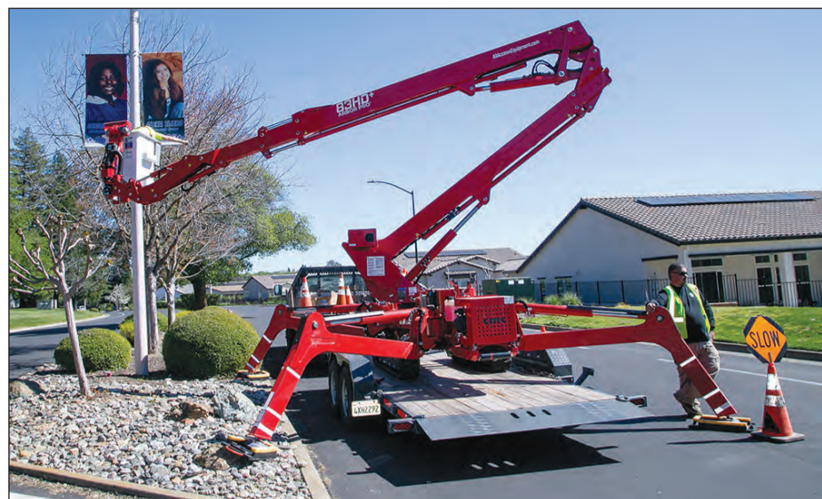
Daniel Esquivel directs traffic while a co-worker installs senior banners from the association's new aerial lift along Murieta Parkway.
