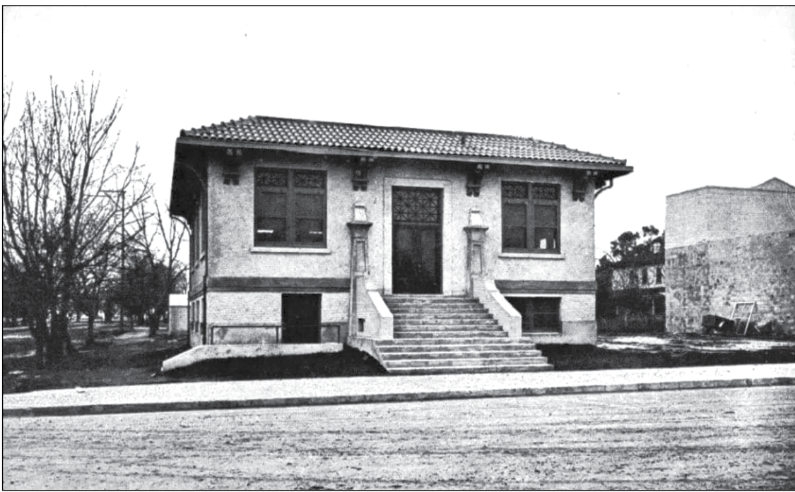
Built in 1916 with support from industrialist Andrew Carnegie, the former Gridley Public Library reflects both a national movement and a local effort driven by community members. Courtesy photo
