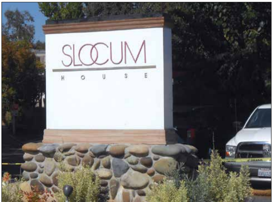
Ongoing renovations of the beloved Slocum House restaurant at 7992 California Ave. in Fair Oaks Village will reflect modern touches with the classic characteristics that have made the Slocum House a historic and treasured local landmark.
