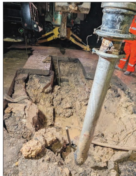
Repair work on Pescado Circle is underway on Jan. 4. Courtesy photo
