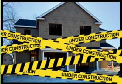
55 & 57 A St. Franklin Under Construction
