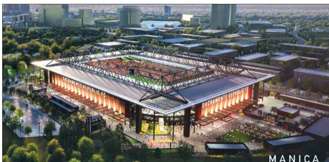
Wilton Rancheria and Sacramento Republic FC have announced that Republic Stadium at The Railyards will be constructed as a 20,000-plus seat soccer-first venue, forgoing the original plans to grow through phased expansion. Photo courtesy of Republic FC/MANICA
