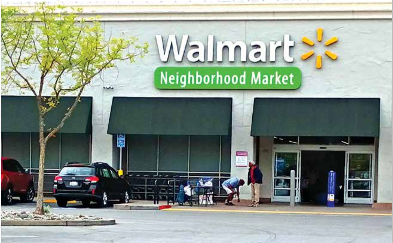
Remodeling work has started on the interior of the Walmart Neighborhood Market grocery store at 6197 Sunrise Blvd. in the MarketPlace in Birdcage. Photo by Thomas J. Sullivan
