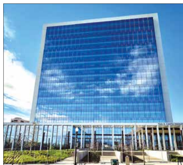
The new Tani G. Cantil-Sakaue Sacramento Superior Courthouse located in the Sacramento Railyards is set to open next month. Photo courtesy of Sacramento County Superior Court
