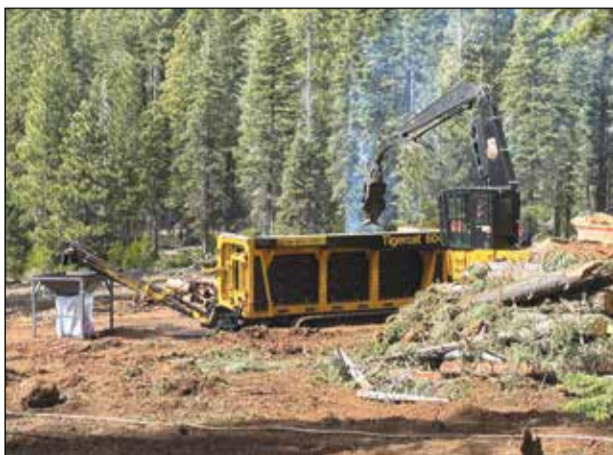
A carbonizer processes wood waste near Jonesville in the Lassen National Forest as part of a PG&E pilot project aimed at reducing hauling and emissions. Photo courtesy of PG&E
