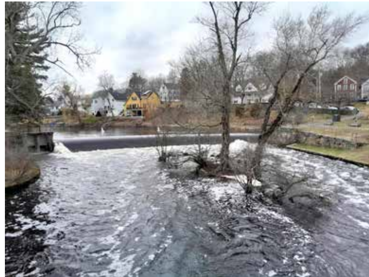
Long an attraction for artists and nature lovers, the Charles River Dam is scheduled to be removed over the summer, as part of a site improvement project. Photo by Maureen Sullivan
