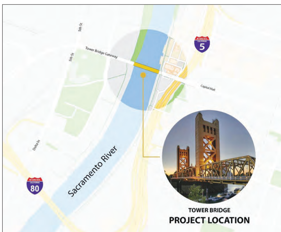
Caltrans recently announced that motorists should expect partial daytime closures on the Tower Bridge (State Route 275) from now until November, with daily one-way intermittent traffic control in place from 7 a.m. to 3 p.m. Image courtesy of Caltrans
