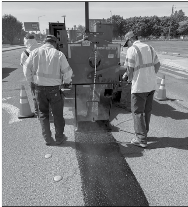
Yuba City Street Maintenance crews apply mastic crack sealing on Gray Avenue as part of a preventative maintenance effort to extend the life of local roads and improve driving conditions. Photo courtesy of the City of Yuba City
