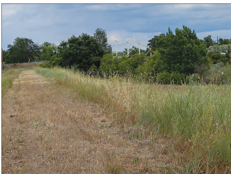
The levee road west of the Cosumnes River is shown with Highway 16 and the Yellow Bridge in the background. Reclamation District 800 plans to repair erosion-damaged riprap on the river side of the levee east of this location. The repair area is not visible in this photograph but is identified on the accompanying map. Photo by Gail Bullen
