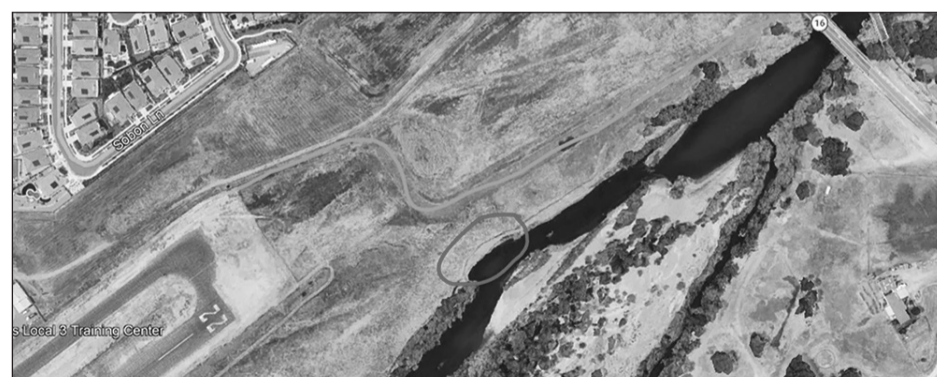
An overhead view shows the location of levee erosion that Reclamation District 800 plans to repair this year. It isn't considered an emergency. Photo courtesy of Reclamation District 800
