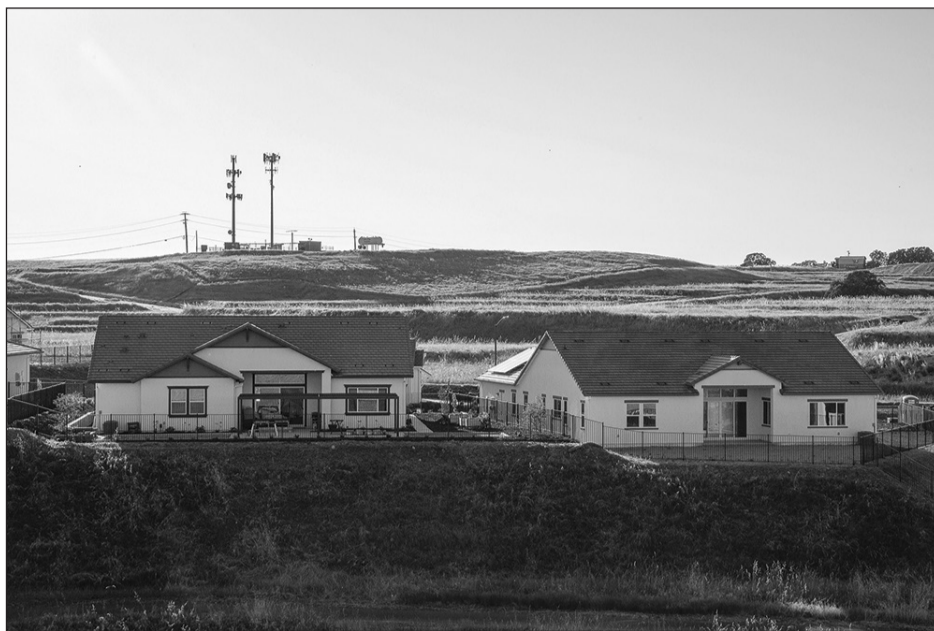
Homes under construction in the first phase of The Residences of Murieta Hills subdivision are shown in the foreground. In the background is the project's second phase, where grading and underground utility work began in 2025. River Canyon Properties alleges uncertainty over future water-meter issuance has delayed further development of the 198-lot subdivision. Photo by Gail Bullen
