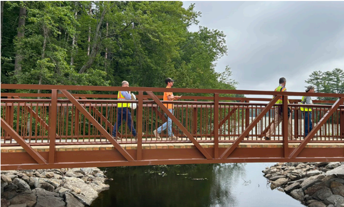
Pedestrian bridge over Singletary Bridge at former Arnold Pond Dam site. Photo supplied by Caleb Slater
