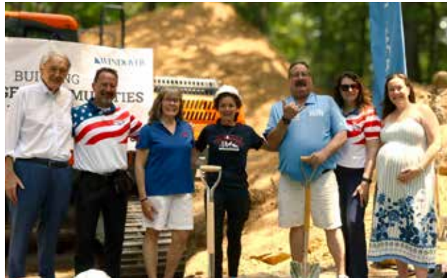
Construction of the MetroWest YMCA Regional Early Learning Center in Ashland officially broke ground last month, with help from federal, state and private funds. Photo supplied by Michael Henrich
