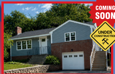
7 Dana Park. Hopedale Coming Soon | Under Construction
