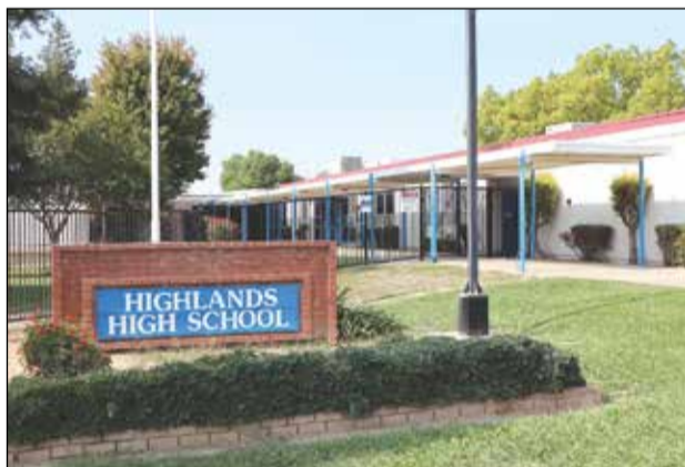
Highlands High School is among the schools undergoing summer projects, with a canopy replacement and gym improvements underway. Photo courtesy of Twin Rivers Unified School District
