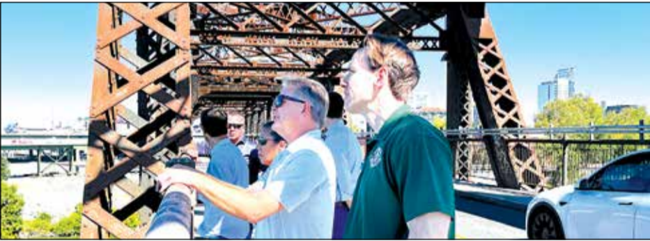
A new bridge will provide a new connection across the Sacramento River between the Sacramento Railyards and the West Sacramento Washington Neighborhood planned developments. Photo courtesy of Office of Kevin Kiley
