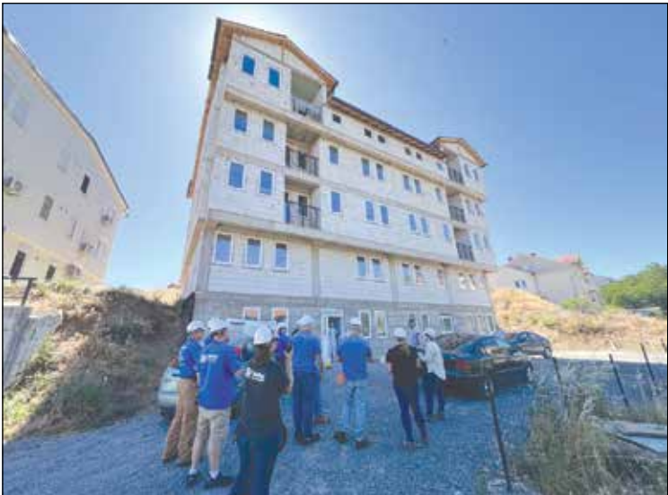
Habitat for Humanity Yuba/Sutter volunteers gather outside a housing project in Veles, North Macedonia, where they helped with construction work, including insulation, plastering, priming, waterproofing, tile installation and drywall. Photo courtesy of Habitat for Humanity Yuba/Sutter
