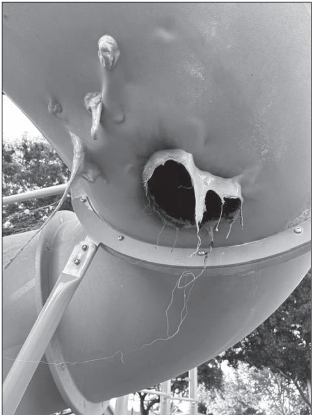
A slide at the Sports Complex Playground has been temporarily closed following an act of vandalism. Photo courtesy of the City of Galt information becomes available regarding repair plans and the reopening of the playground feature.
