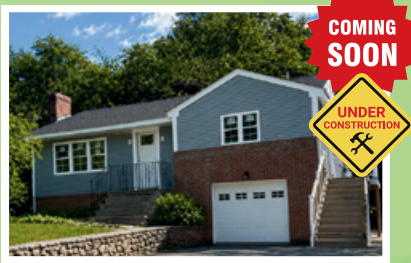
7 Dana Park. Hopedale Coming Soon | Under Construction
