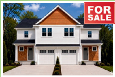
57 A St. Franklin For Sale - Under Construction
