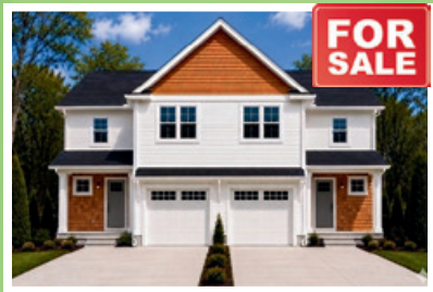
55 A St. Franklin For Sale - Under Construction
