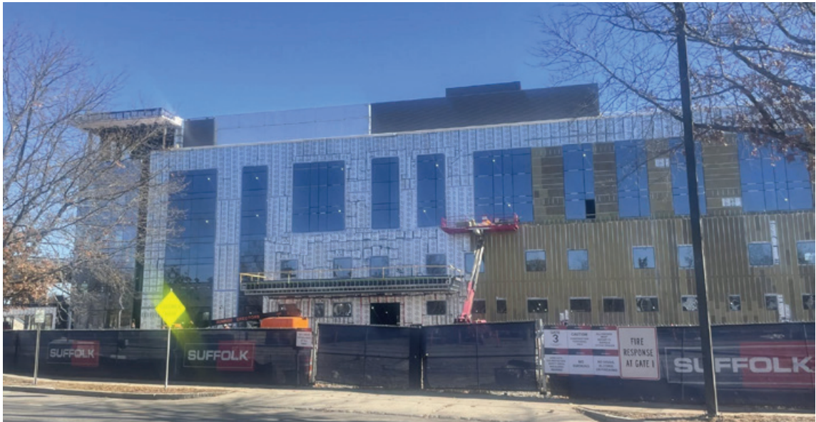
The replacement Norwood Hospital is shown under construction in February 2025. Construction was later halted, and the future of the site remains the subject of legislative action. (Photo courtesy of Finish Norwood Hospital/Facebook.)
