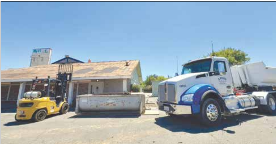
A dump truck, construction bin and forklift sit outside the Tri-Counties Community Center during demolition work July 16. Exterior renovations are expected to continue through August.
