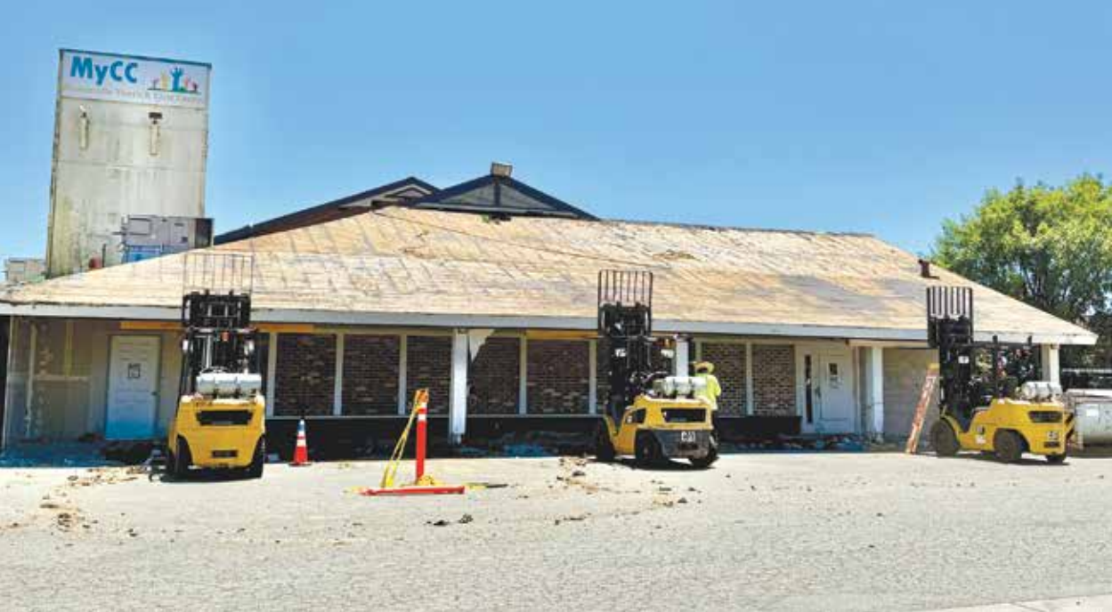
The roof, siding and portions of the sidewalk are stripped from the Tri-Counties Community Center in Marysville on Thursday, July 16, as exterior renovations move forward.
