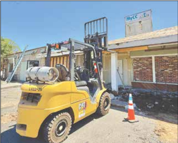
Construction equipment stands outside the Tri-Counties Community Center on July 16 as crews remove damaged exterior materials and prepare the Marysville building for repairs.
