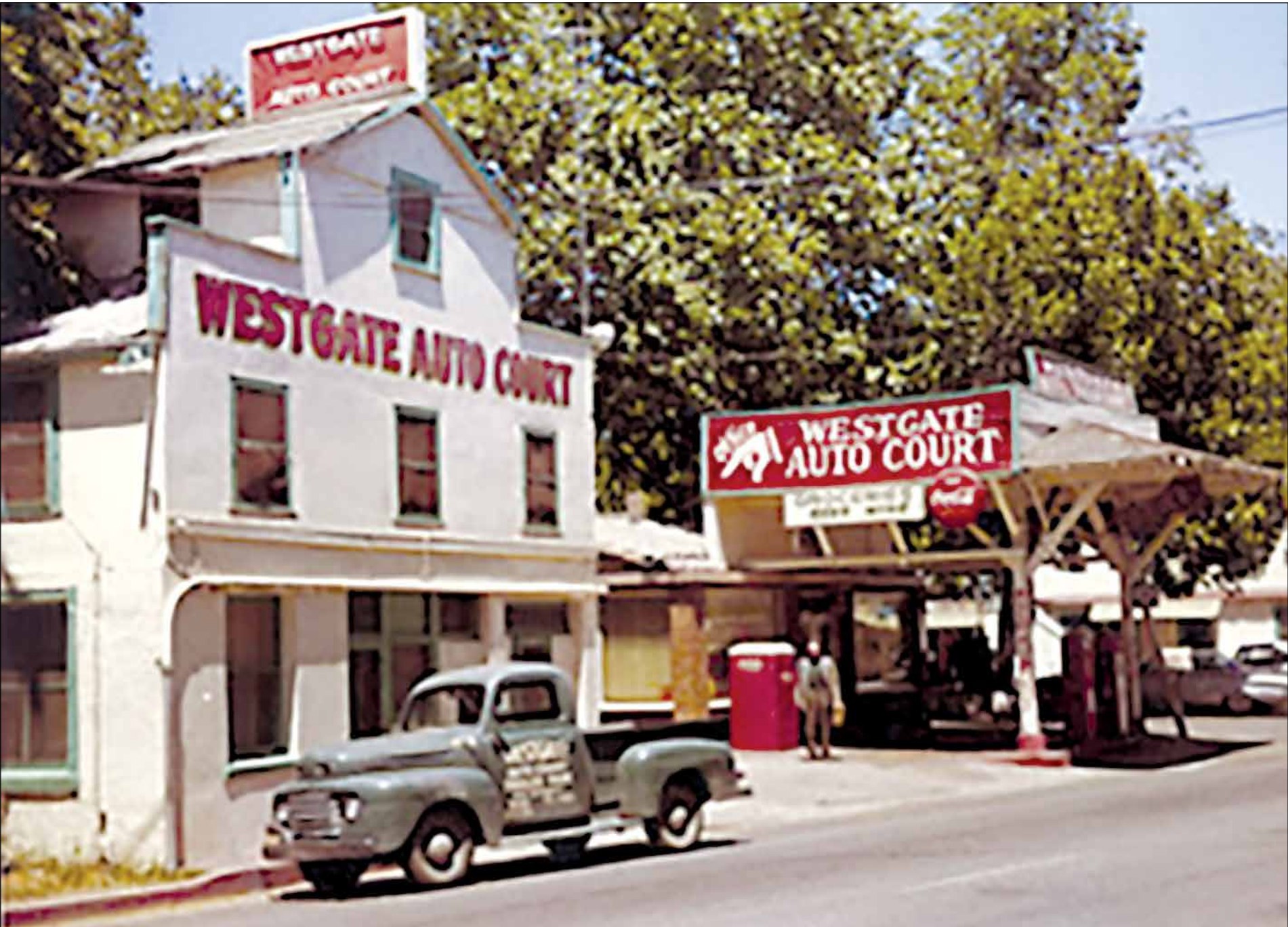
The Westgate Auto Court and Trailer Park was one of several auto courts that began operation in West Sacramento in the 1920s. Photo courtesy of Susan Curtis Willats
