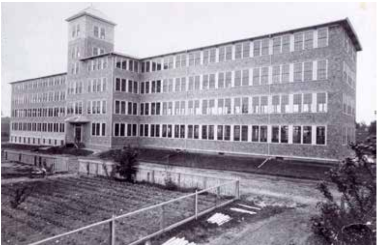
Construction of the Huckins, Temple & Wood Shoe Factory. 7 & 9 Charles Street, opposite 53 Depot Street. Courtesy photos
