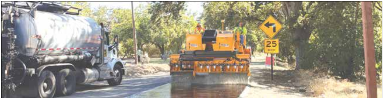
In July, SacDOT launched a unique Chip Seal program to provide a more economical approach to repairing damaged roads. Photo courtesy of Sacramento County
