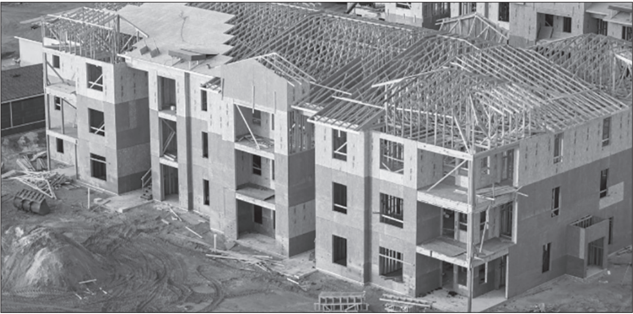
The county will allow eligible affordable housing projects to receive offsets for development impact fees for three separate parks districts. Photo courtesy of Sacramento County
