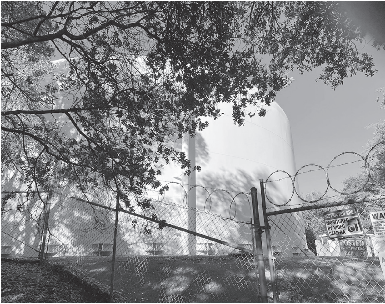
The Rio Oso water storage tank is at the center of a renewed debate over the construction of a third storage tank after district staff said it will require major rehabilitation in about 2½ years. File photo
