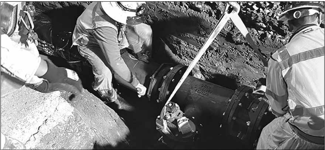
The Arden Service Area Pipe and Meter Installation Project spanned 10 years, and SCWA installed approximately 38 miles of new water distribution pipelines and more than 3,000 new water meters. Photo courtesy of Sacramento County
