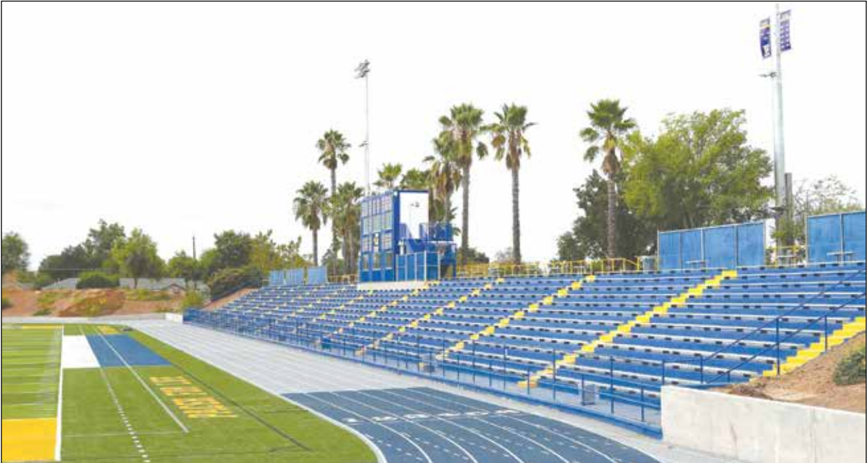
Stadium upgrades include an all-weather track, turf improvements and new press box. Photo courtesy of Twin Rivers Unified School District
