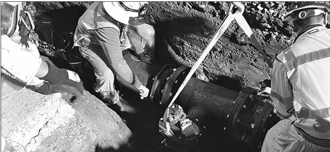
The Arden Service Area Pipe and Meter Installation Project spanned 10 years, and SCWA installed approximately 38 miles of new water distribution pipelines and more than 3,000 new water meters. Photo courtesy of Sacramento County
