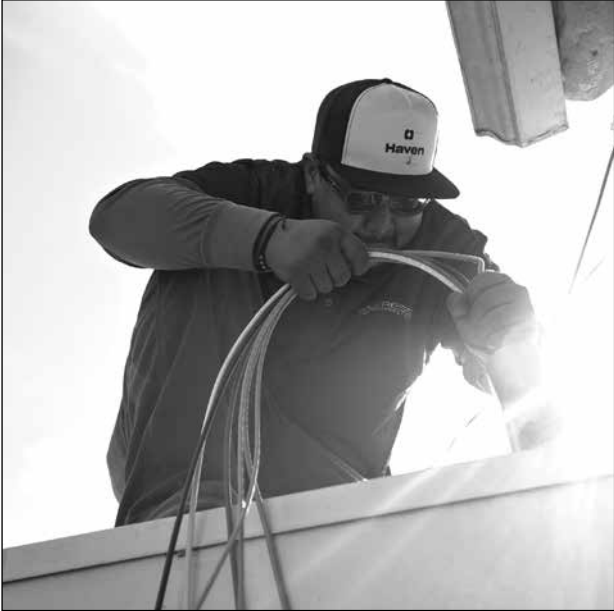
Haven Energy, the No. 1 SGIP developer in California, is working to connect income-qualified California homeowners with nearly $8.7 million in remaining state funding that can provide households with home battery systems at no cost.
