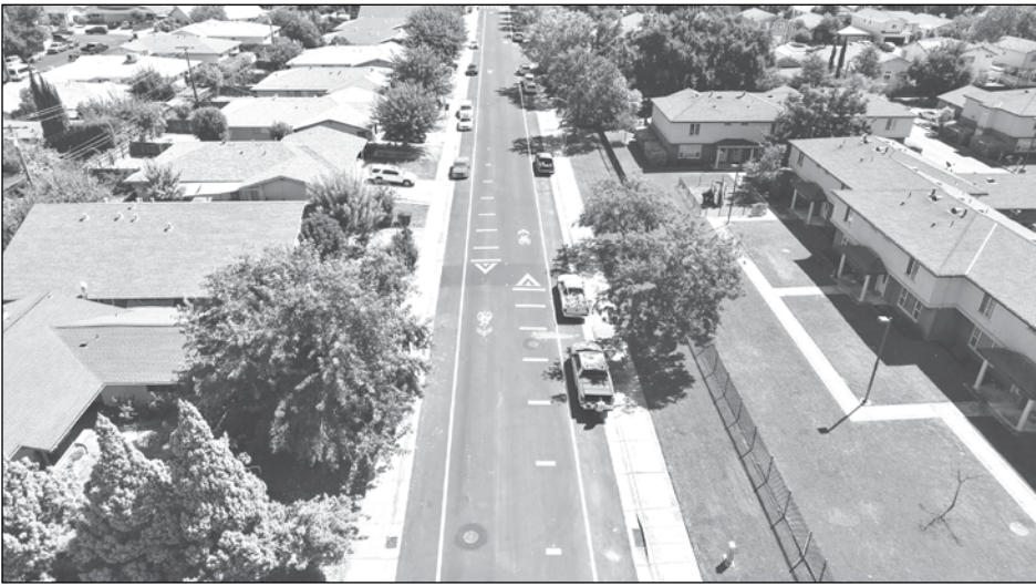
Streets are being rehabilitated with resurfaced roadways, drainage improvements and high-visibility roadway markings. Photo courtesy of the City of Rancho Cordova
