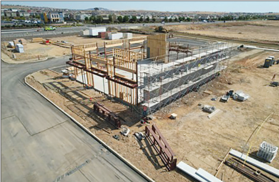
JP Masonry is working on Alder Creek Marketplace in Folsom. Photo courtesy of JP Masonry
