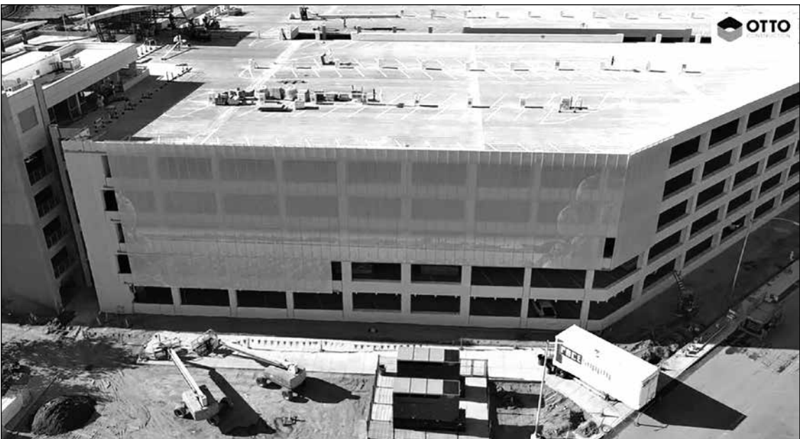
SMF will adjust public parking rates when the new Parking Garage 2 opens later this year. Photo courtesy of Sacramento International Airport/Otto Construction
