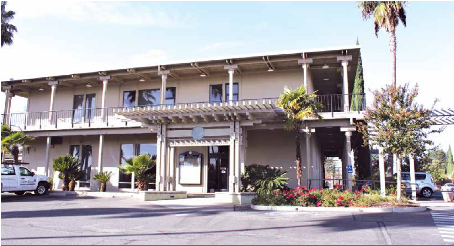
Cave reflected with pride at the city’s steady growth and her own first days as an entry-level office assistant walking through the front doors of the old City Hall building at Fountain Square in the year 2000. Today, a modernized Dignity Health building stands in its place. Photo courtesy of the City of Citrus Heights
