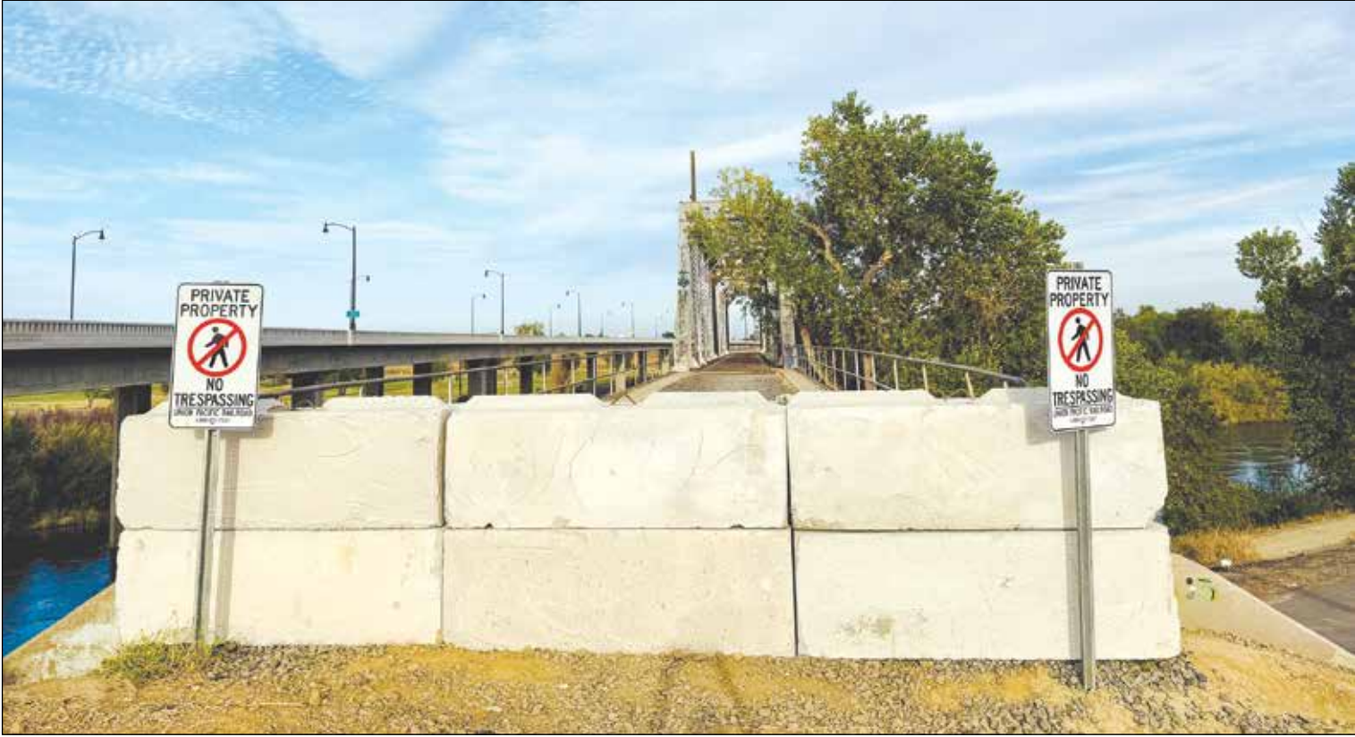
Concrete barriers and Union Pacific “Private Property/No Trespassing” signs now block the Yuba City entrance to the former railroad trestle spanning the Feather River. The new barriers mark a significant change from conditions observed by the Territorial Dispatch before Alina Lynn’s Aug. 9 death.
