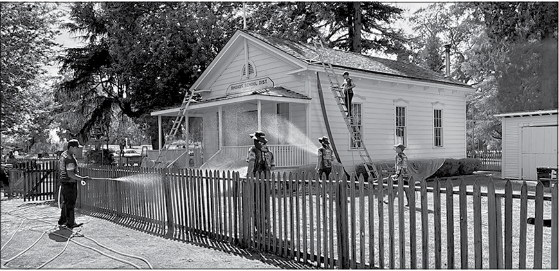
Rhoads School – Workers with No Moss Softwash clean the Rhoads School to get it ready for the Oct. 10 celebration. Photo courtesy of No Moss Softwash
