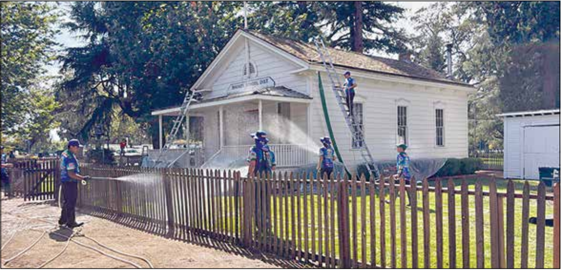
Rhoads School – Workers with No Moss Softwash clean the Rhoads School to get it ready for the Oct. 10 celebration. Photo courtesy of No Moss Softwash
